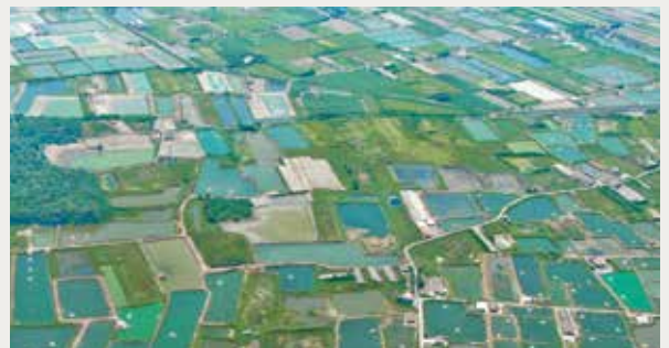
養殖輸水工程 Water Supply engineering
