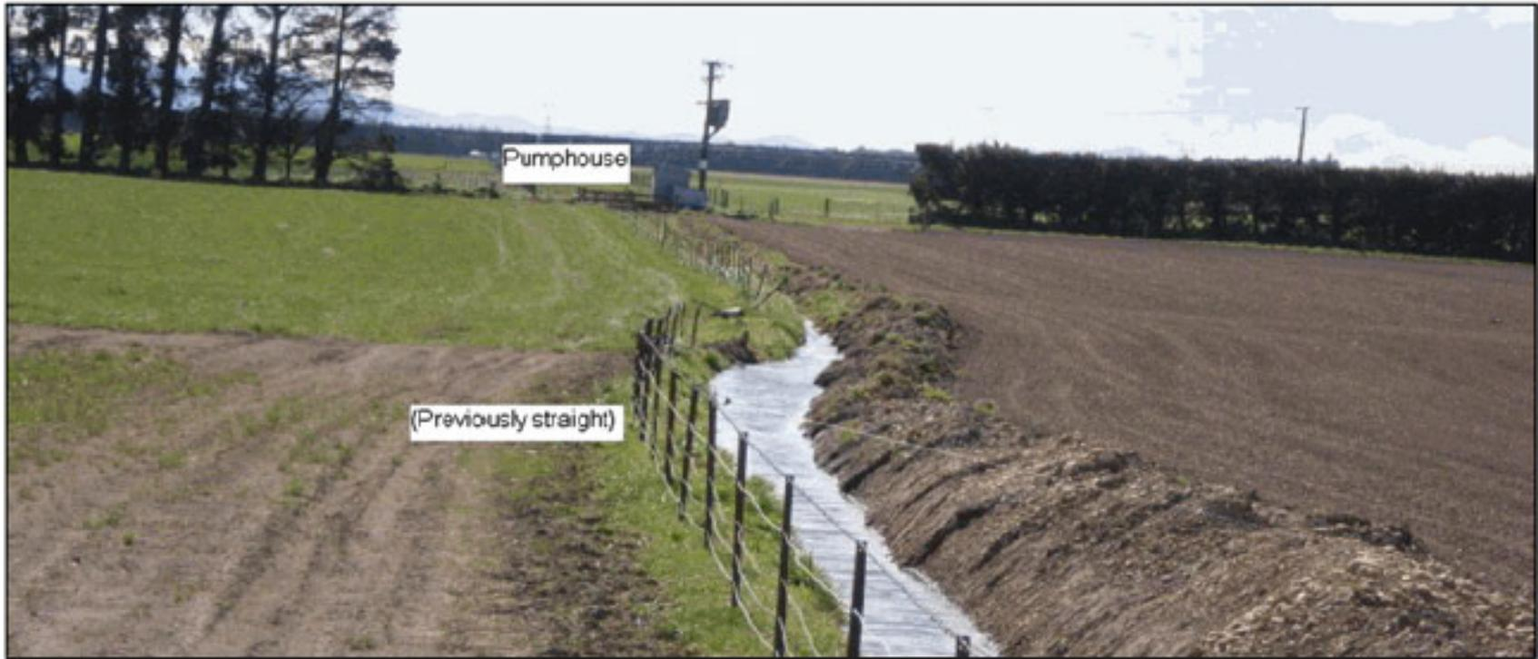
1. Effects of fault rupture on previously straight fence and water race (Photo: Survus Consultants)
