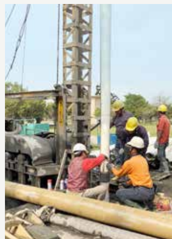
鑿井工程 Well drilling engineering
