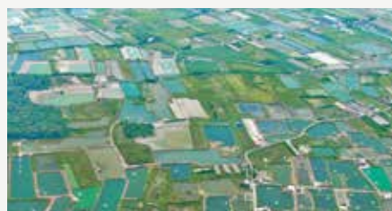
養殖輸水工程 Water Supply engineering
