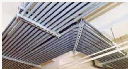
建築工程 Architectural engineering
