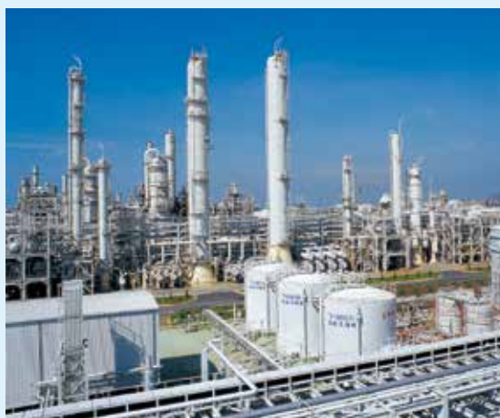
工廠排水配管 Petrochemical plant
