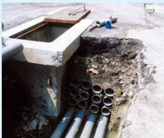
固網通訊工程 Cable net-work communication engineering
